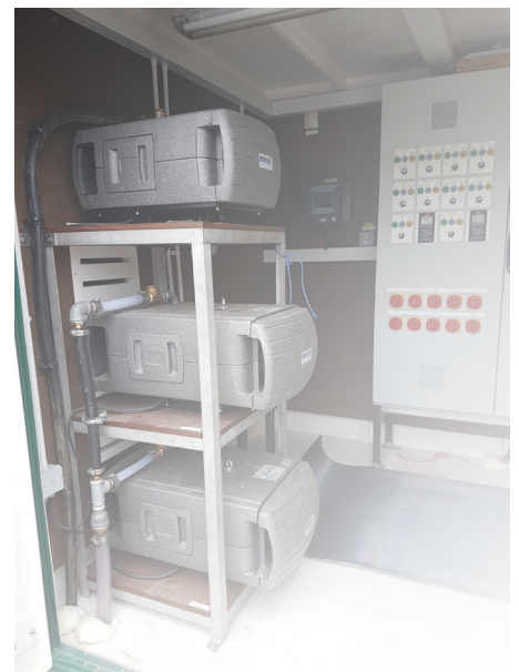
Photographed: BECKER DT compressors housed in soundproof enclosures
